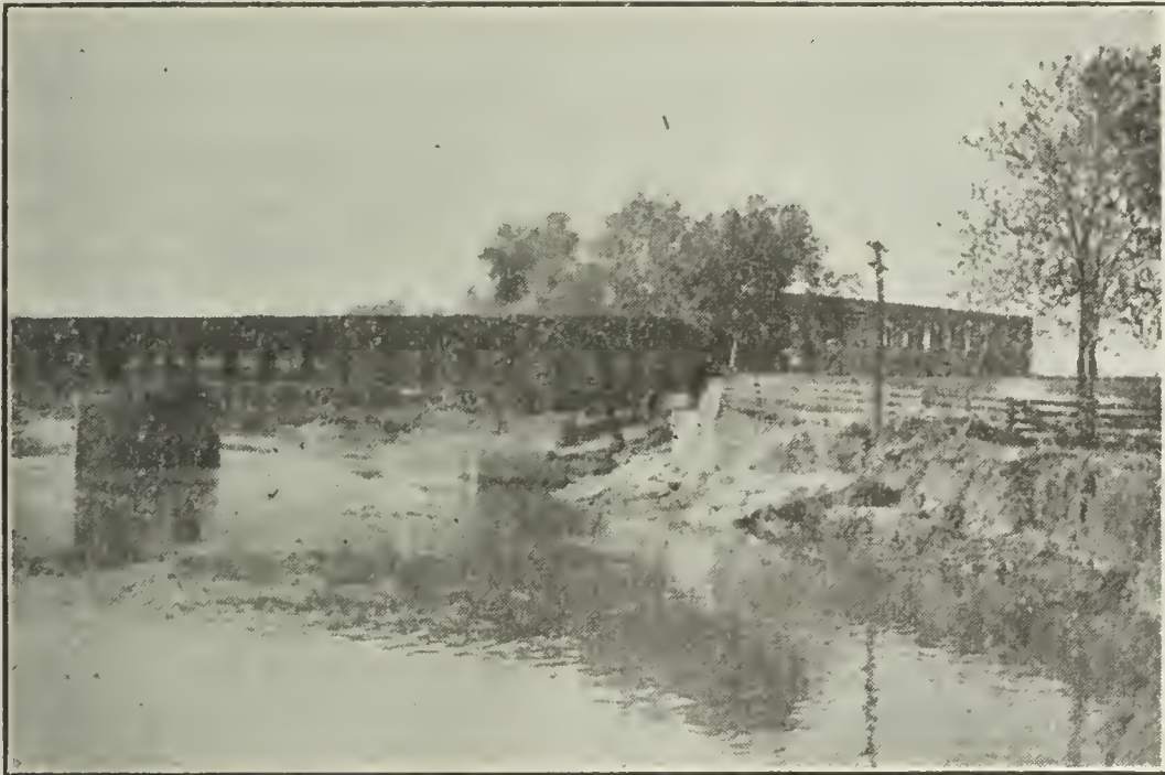
B. Bridge, Looking Up Stream.
